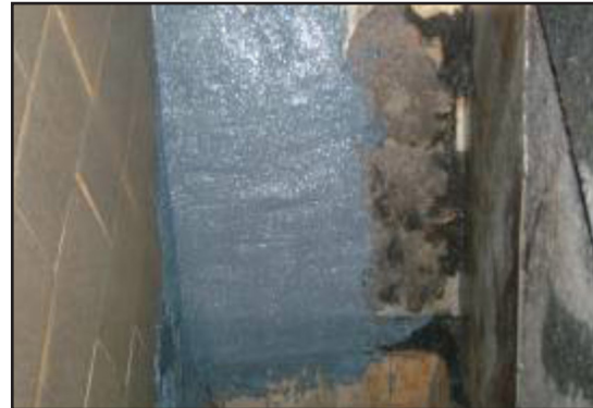
Application of ARC BX5
